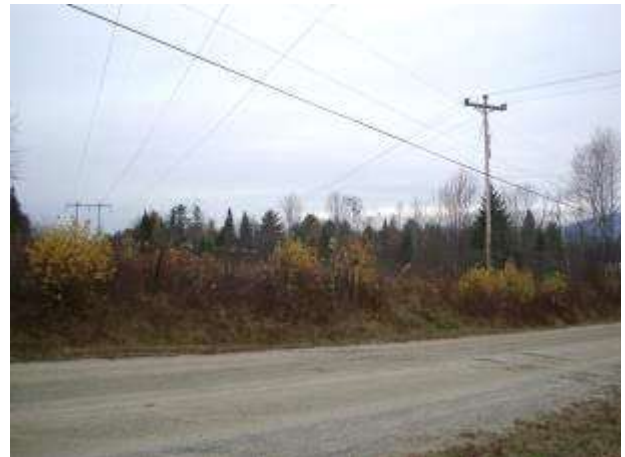
Looking northerly across Wesson Road. The existing line will be moved to the right; the new line will be in the locus of the currently existing line.
