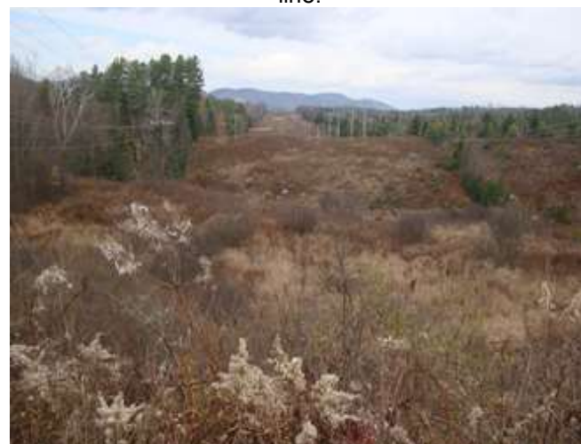
View looking northerly from the vicinity of Pole 686. The new line will be between the existing lines.
