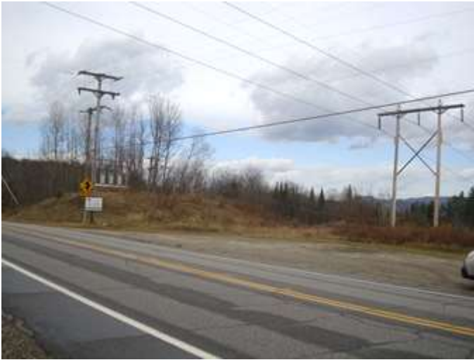
View northerly across Route 301; the new line will be to the left of the existing line.
