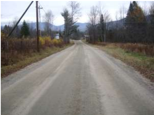
Looking westerly along Wesson Road under the existing ROW.
