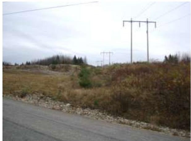
Looking westerly from Bell Hill Road.
