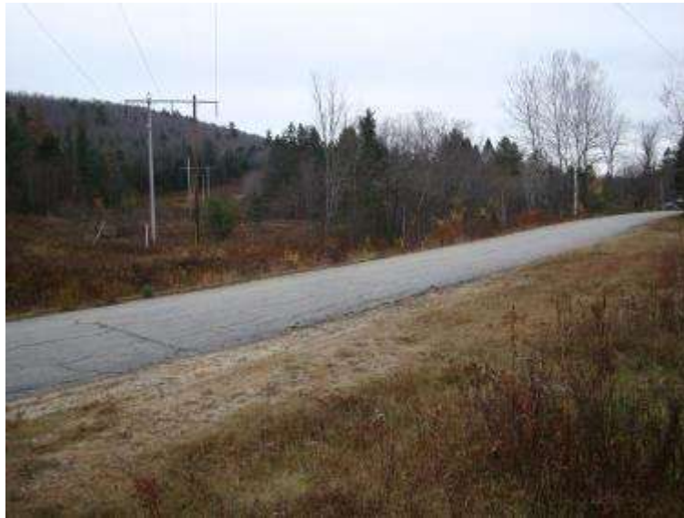
Looking westerly across Potter Road.; new line will be to the right of the existing.
