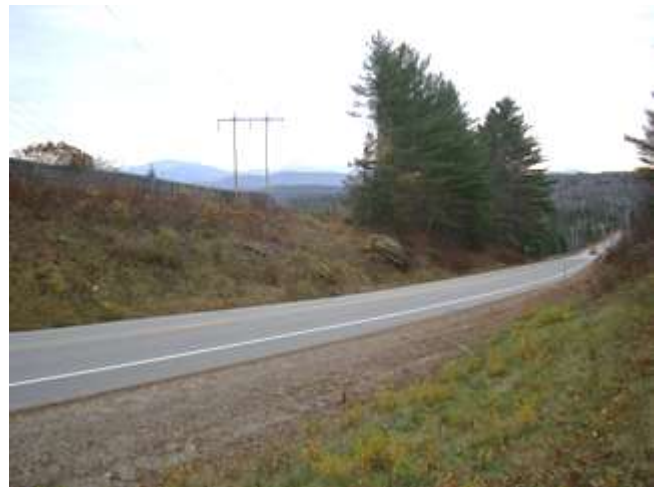
Looking southerly across Route 116. There are some residences in the vicinity on Route 116. The new line will be in the same locus as the existing one, which will be moved.
