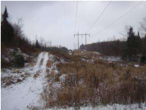
Looking easterly from the private road off Route 110.
