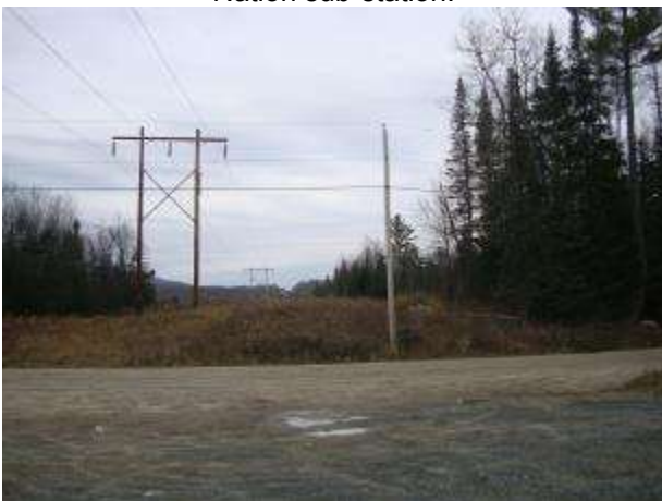
Looking northerly across Page Hill Road; the new line will be left of the existing.
