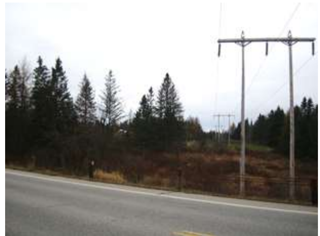
Looking southerly across Route 2. The new line will be in about the same locus as the existing which will be moved.
