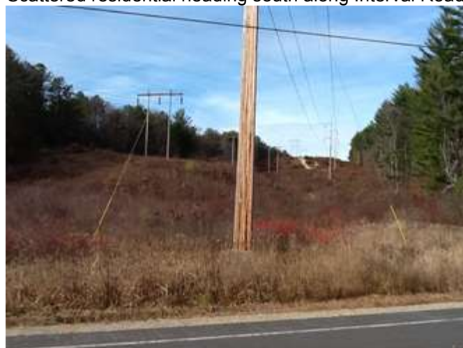
West Road crossing.
