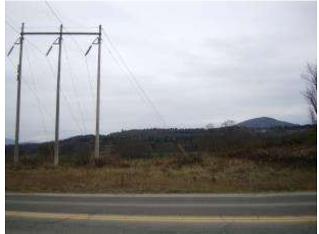
Looking southerly across North Road; new line will be just to the right of the existing.
