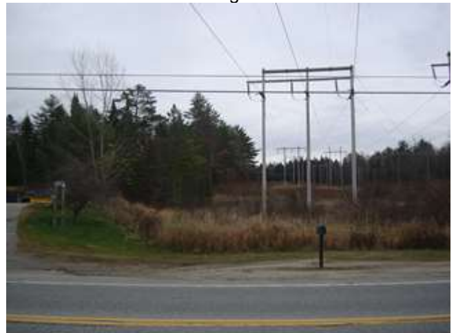
Looking easterly across Route 3—a more developed neighborhood. The new line will be along the left side.
