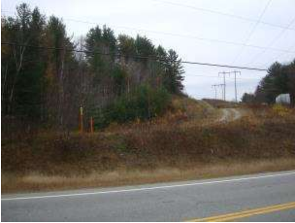
Looking easterly across Route 110; new line will be on the left of existing.
