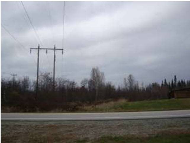
Looking northwesterly across Route 116 near Hatfield Drive; the locus of the new line will be just to the right of the existing line.
