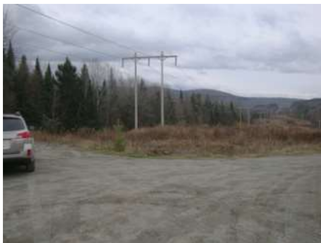
Looking southerly from the end of Stoney Acres Drive. The new line will be to the right of existing line.
