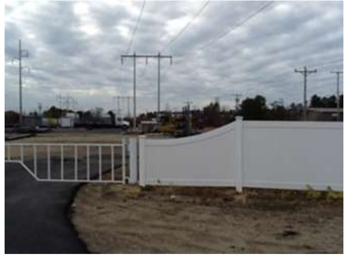
Regional Drive Both north and south the easement crosses through industrial storage yards.
