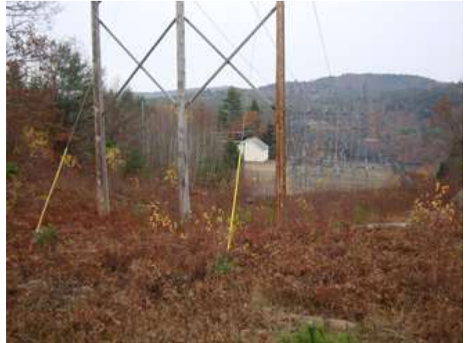
Looking northerly Pemigewasset s/s in the vicinity of new pole #1177 south of Old Bristol Road.
