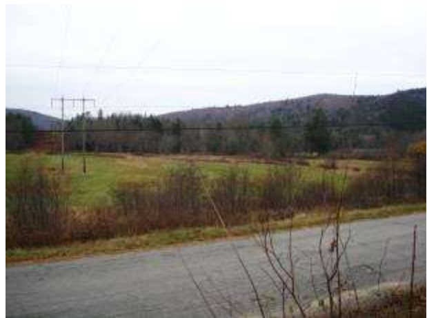
Looking westerly across Northside Road across open field; new line will be on the right of existing.
