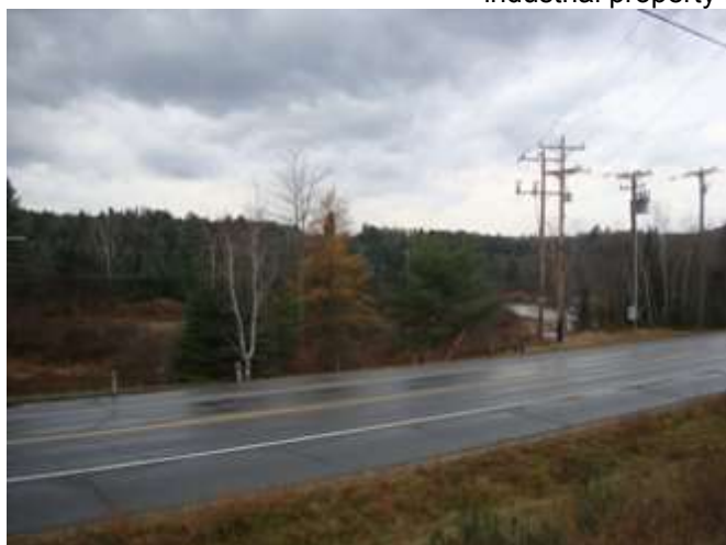
Looking southwesterly across Route 3 and across river through undeveloped woodland. The new line will be between the existing lines.
