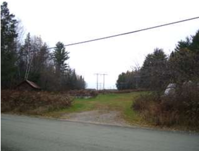
Looking northerly across Nutting Road; the new line will be in the same locus as the existing one which will be moved.
