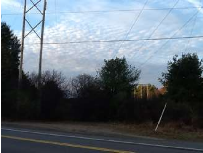
Portsmouth Street Concord crossing I-393
