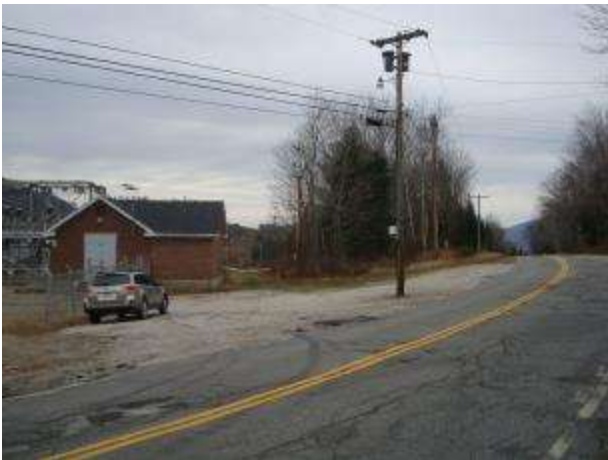
Looking southwesterly across Lost Nation Road; new line will go around on the right of the Lost Nation sub-station.
