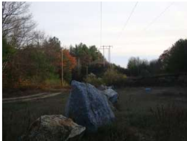
Looking southerly from the vicinity of Pole 113 across brook into New Hampton. New line will be to the right of the existing.
