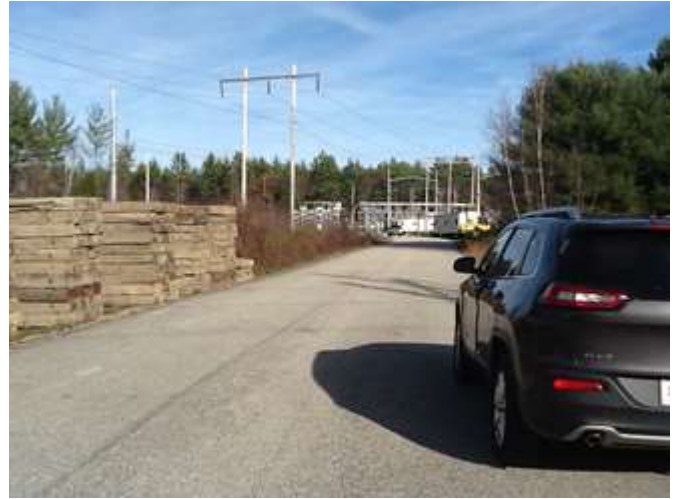
Farmwood Road showing utility transfer station
