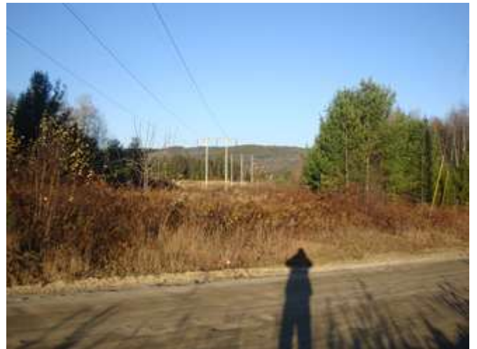
Looking northeasterly across Abell Road; the new line and sand pit is located to the right.
